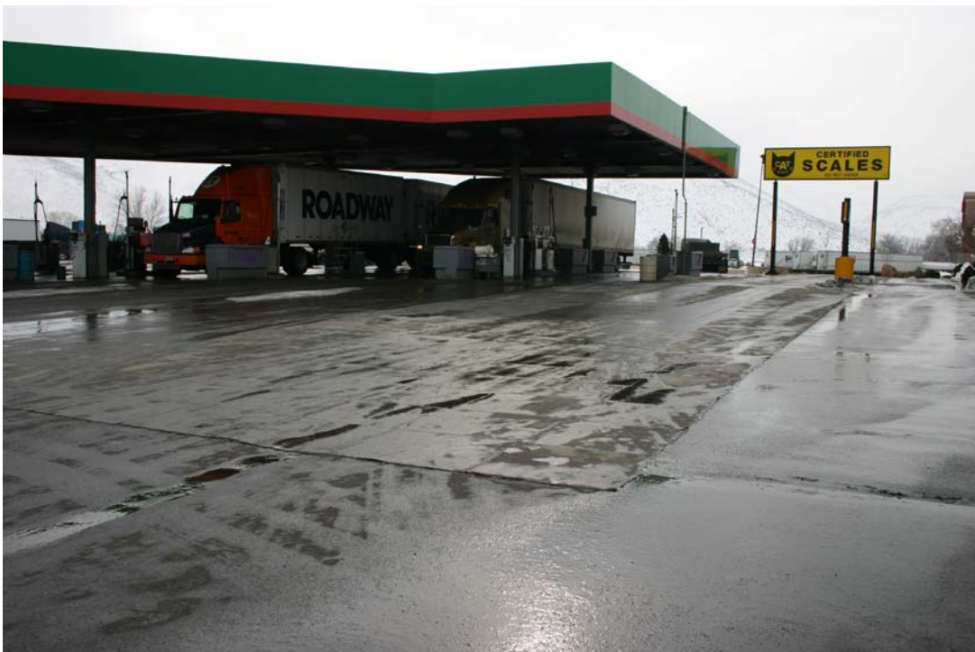
Photograph E Alamo Truck Stop – UTW extends from scale and from pump island adjacent to scale
